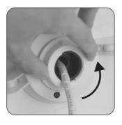
1. Unscrew nut from main unit and slide down cable.
